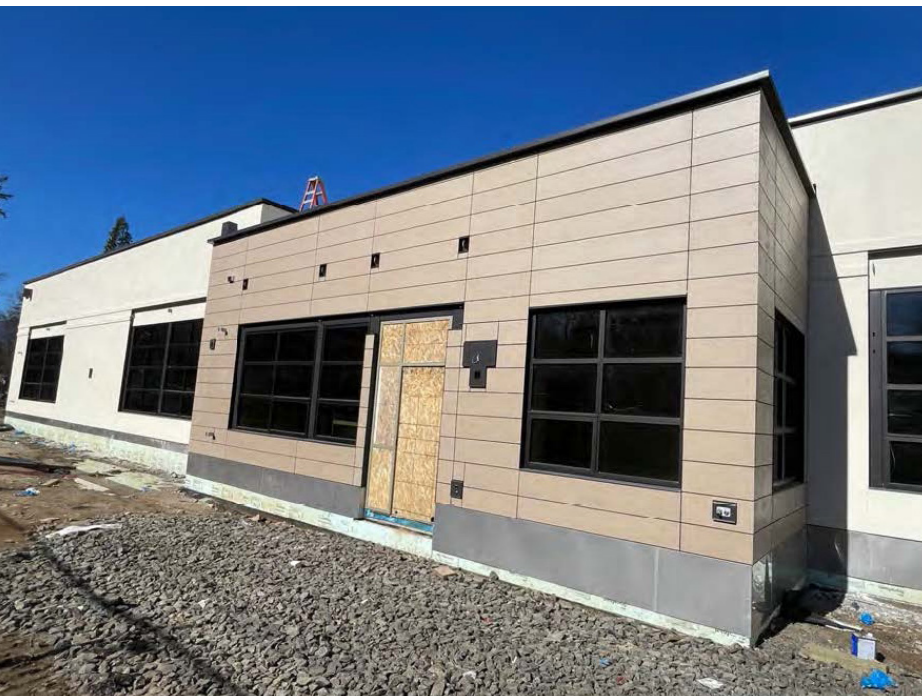
EXTERIOR CEMBRIT CLADDING AND NEW STUCCO AT WALKER ELEMENTARY SCHOOL ADDITION
