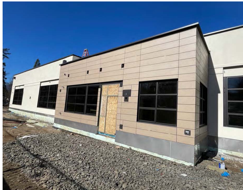
EXTERIOR CEMBRIT CLADDING AND NEW STUCCO AT WALKER ELEMENTARY SCHOOL ADDITION
