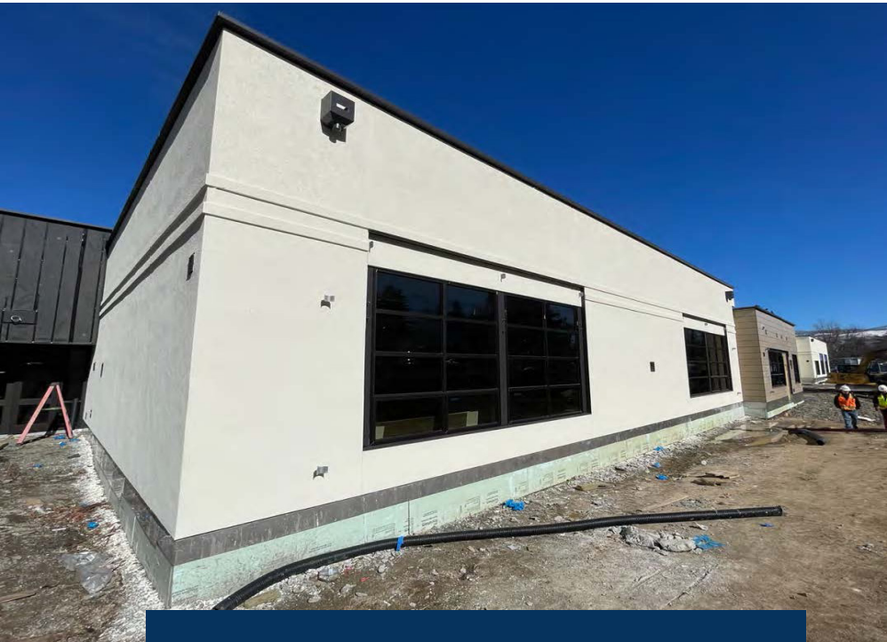
EXTERIOR CEMBRIT CLADDING AND NEW STUCCO ON THE SOUTH SIDE OF THE BUILDING
