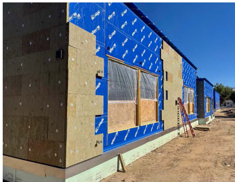
EXTERIOR INSULATION
