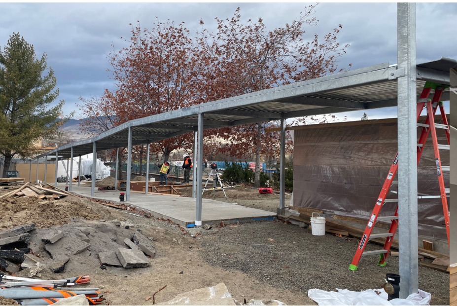
STRUCTURAL STEEL AT COURTYARD COVERED WALKWAYS
