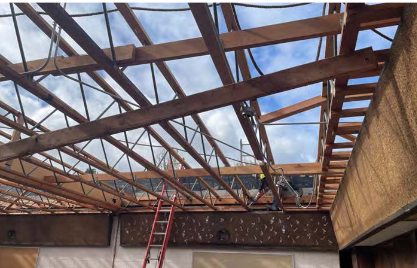
REPLACEMENT OF SELECT STRUCTURAL MEMBERS AND ROOF AT MUSIC ROOM / GYM
