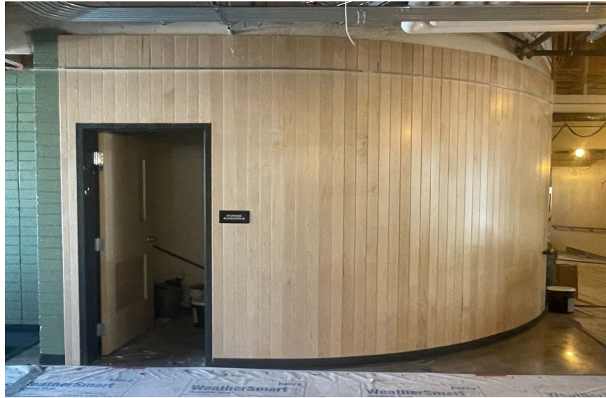
Tongue and Groove Wall Covering at the Admin Area of TRAILS
