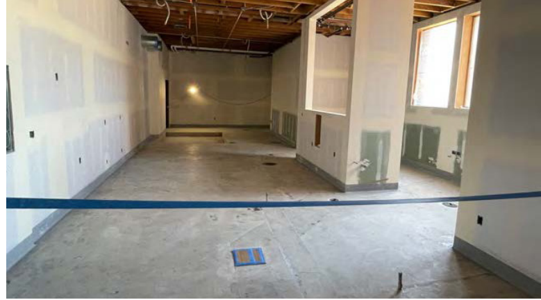
COMPLETION OF SHEETROCK INSTALLATION AT CAFETERIA AND KITCHEN AREAS
