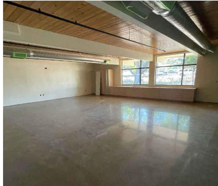
POLISHED CONCRETE FLOORS AND CASEWORK
