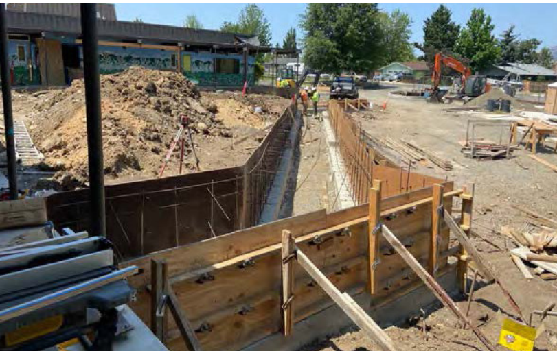
FRONT ENTRY WAY ADA RAMP BEING FORMED
