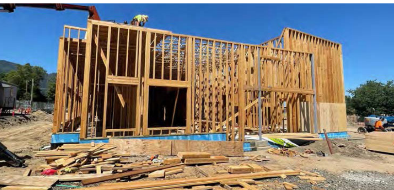
EXTERIOR ELEVATION VIEWS OF ADDITION DEPICTING COMPLETION OF FRAMING/SHEATHING AND FOUNDATION INSULATION
