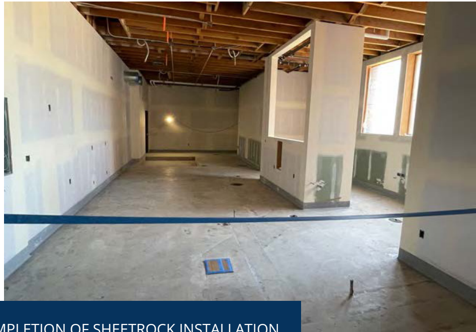
COMPLETION OF SHEETROCK INSTALLATION AT CAFETERIA AND KITCHEN AREAS
