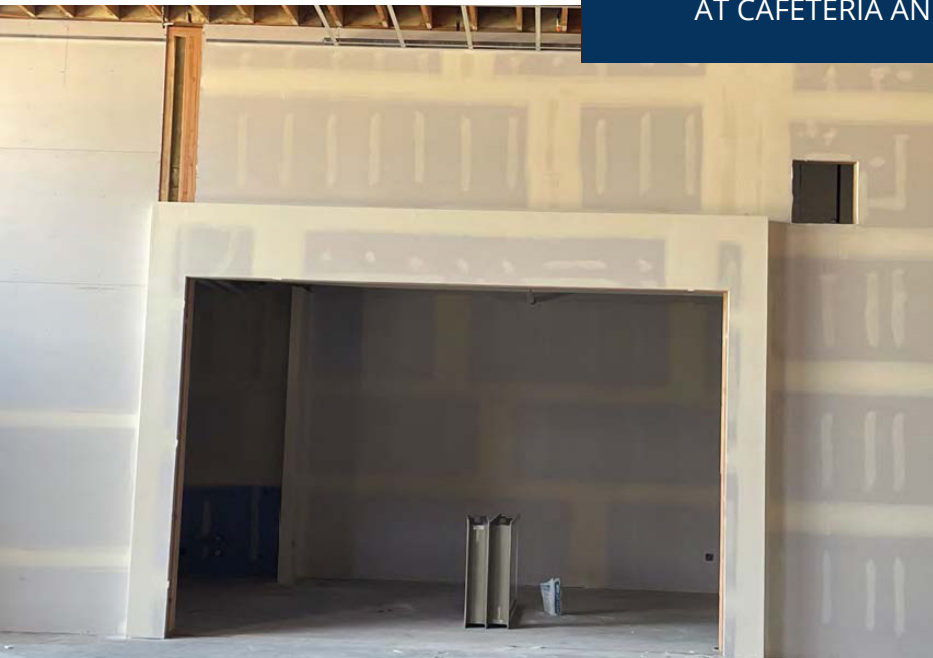
COMPLETION OF SHEETROCK INSTALLATION AT CAFETERIA AND KITCHEN AREAS
