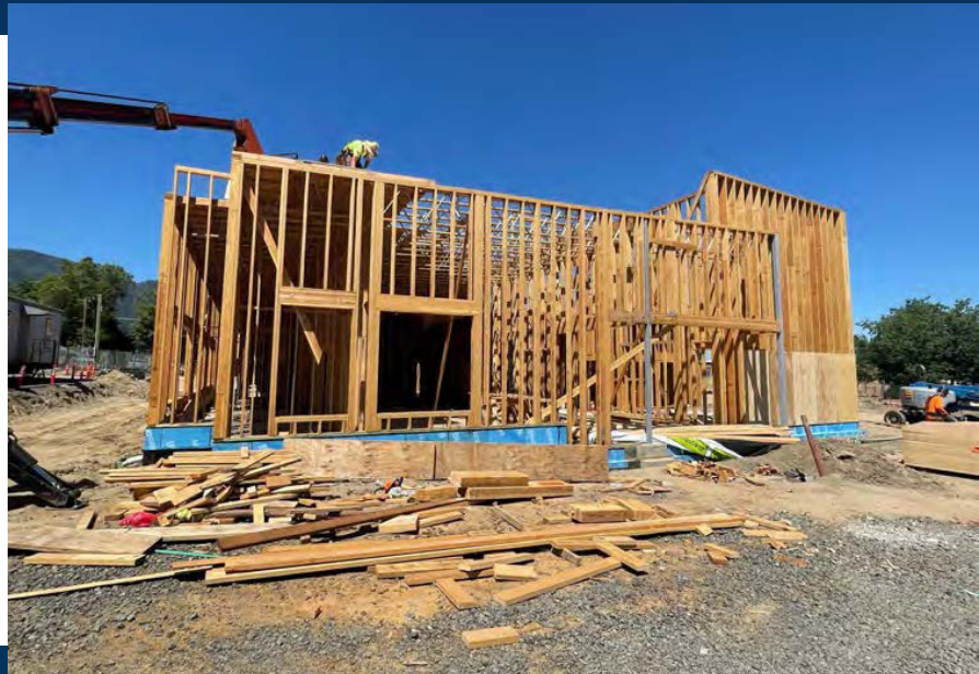
EXTERIOR ELEVATION VIEWS OF ADDITION DEPICTING COMPLETION OF FRAMING/SHEATHING AND FOUNDATION INSULATION
