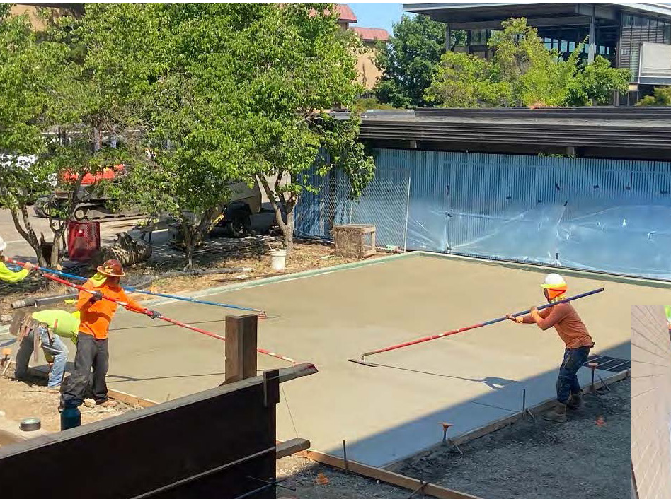
SUNKEN PLAZA FILLED IN AND GETTING CONCRETE FINISHED
