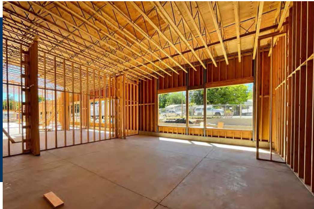
FRAMING AND STRUCTURAL STEEL AT THE ADDITION
