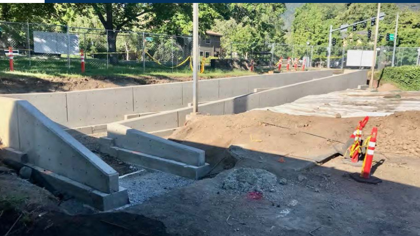
CONCRETE WALLS AND FOOTINGS AT SISKIYOU RAMP
