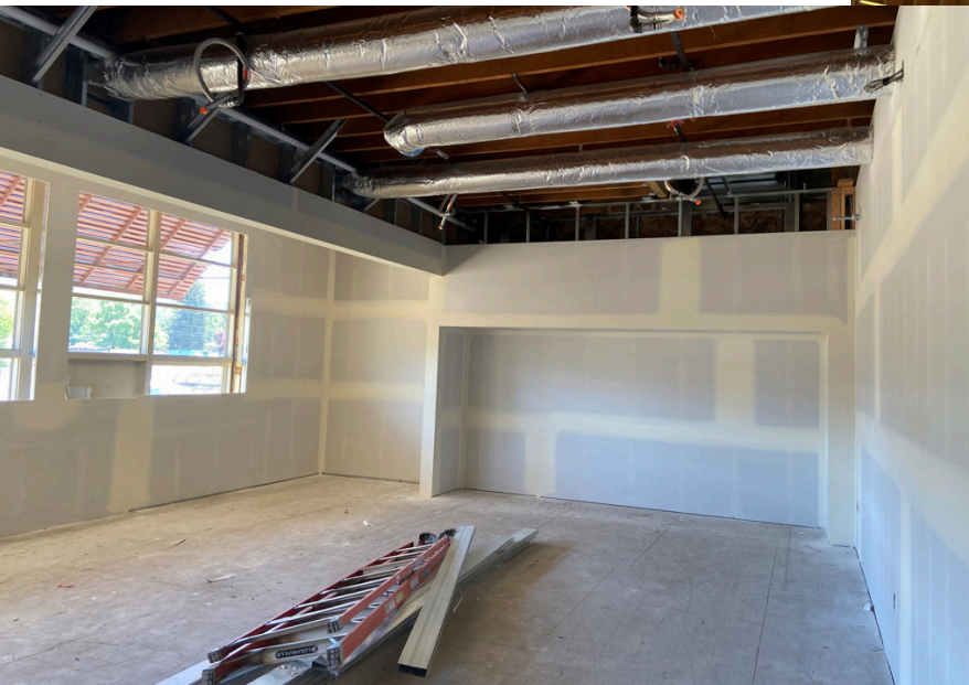
DRYWALL INSTALLATION IN EXISTING CLASSROOM
