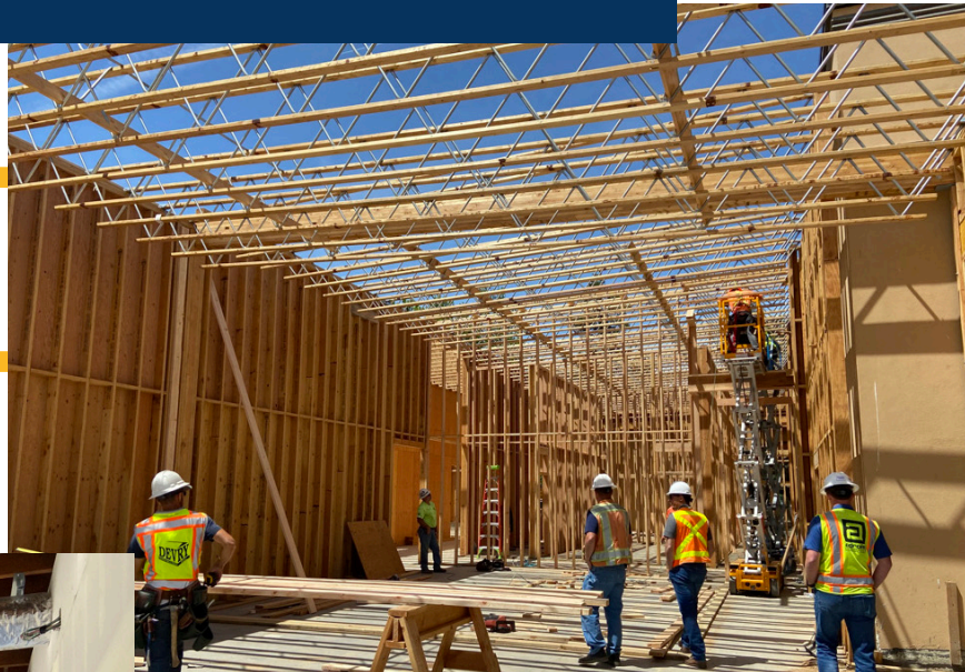
FRAMING AND STRUCTURAL STEEL AT THE NEW ADDITION
