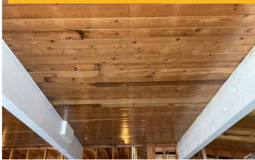
JMOS CEILINGS CLEANED AND SEALED
