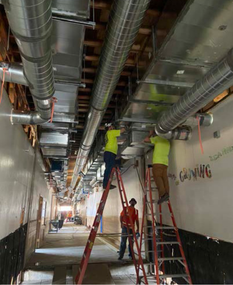
PRESSURE TESTING THE NEW MECHANICAL DUCTING
