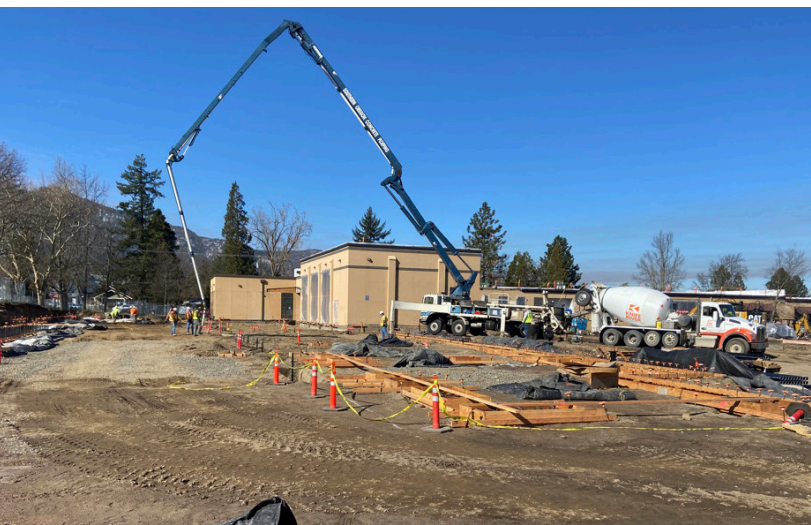
POURING THE CONCRETE NEW ADDITION FOOTINGS
