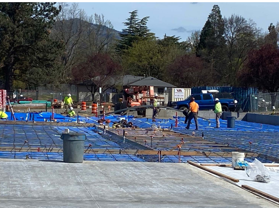
BUILDING SLAB PREPARATION AT WALKER ELEMENTARY SCHOOL NEW ADDITION
