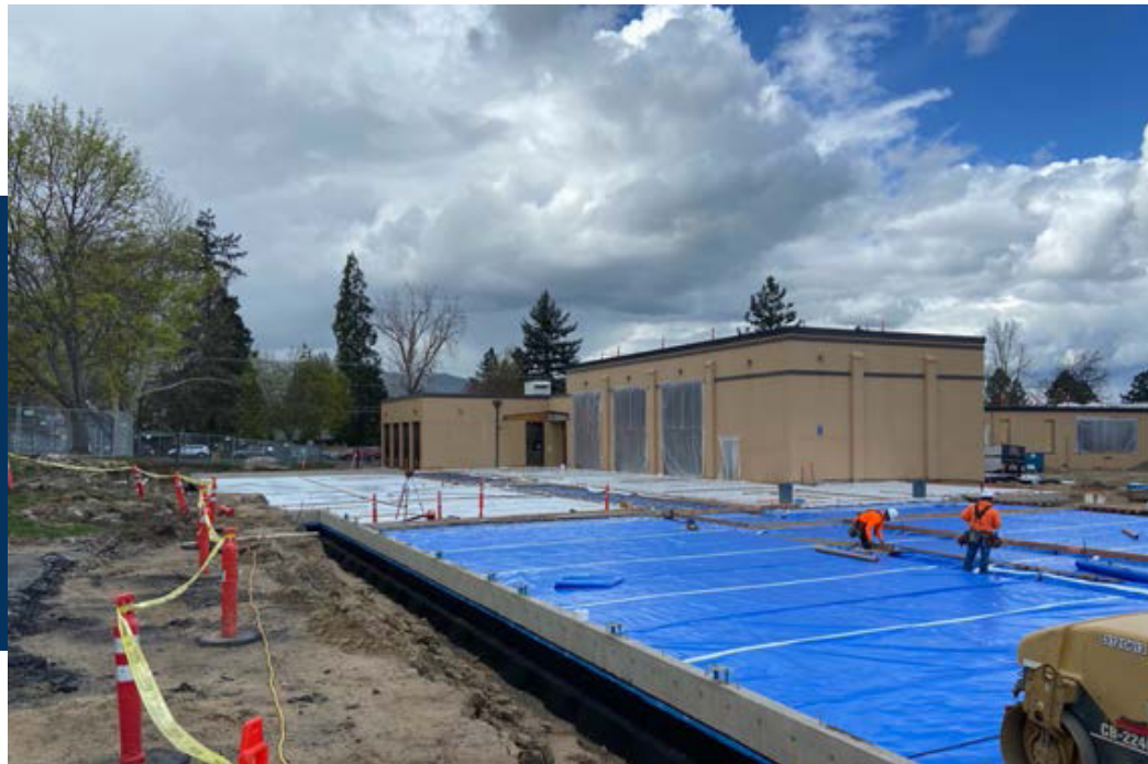
NEW ADDITION CONCRETE PAD PREPARATION
