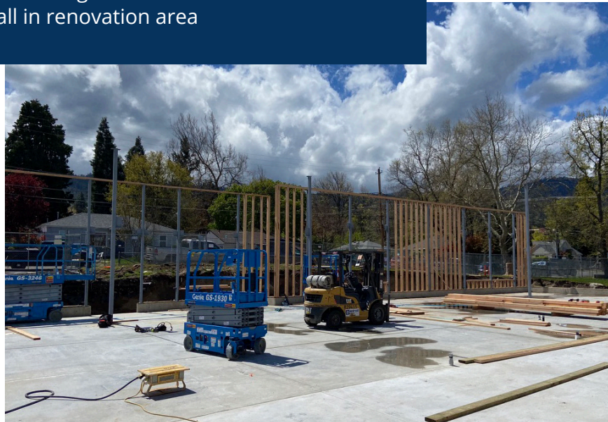
BEGINNING OF THE NEW ADDITION WOOD AND STEEL FRAMING
