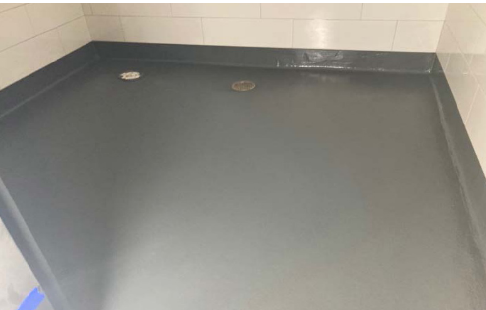
EPOXY FLOOR FINISH IN THE RESTROOMS
