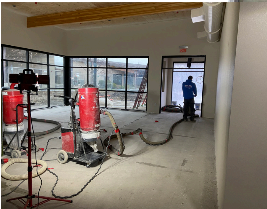
POLISHING THE CONCRETE FLOORS
