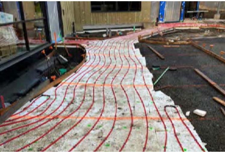
HYDRONIC SNOW MELT LINES THAT WILL BE UNDER
