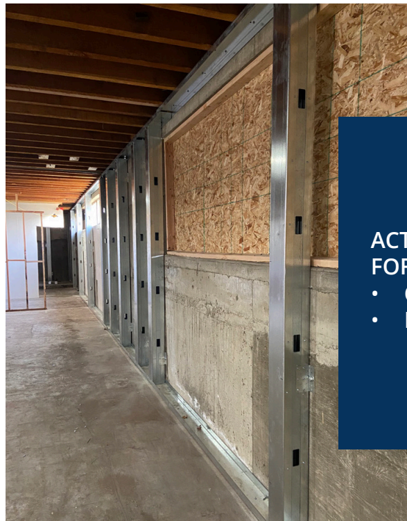
INSTALLATION OF SEISMIC BRACING
