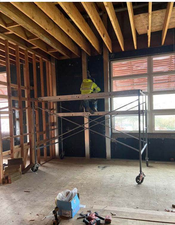
INSTALLATION OF SEISMIC BRACING
