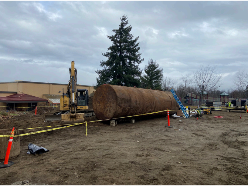
REMOVAL OF THE UNDERGROUND FUEL TANK
