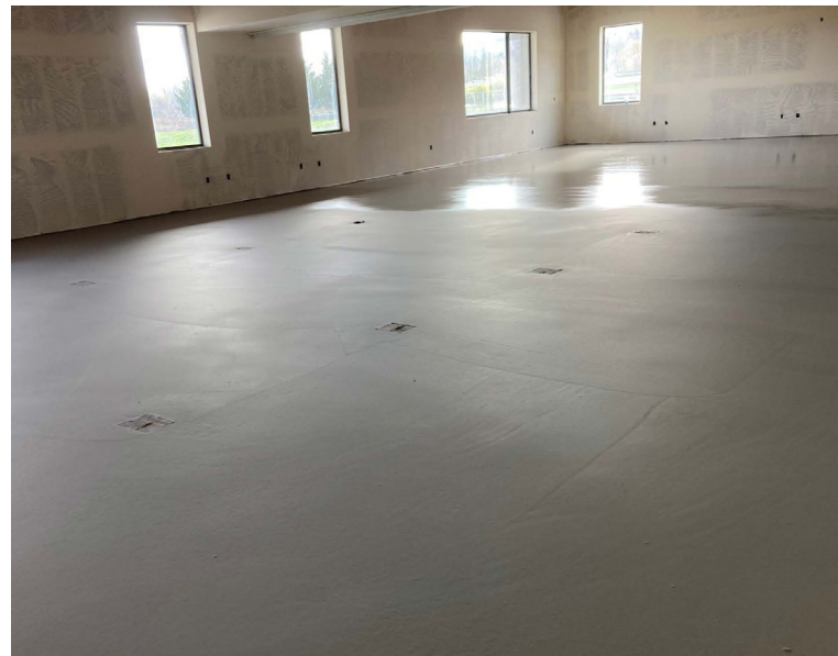
GYPCRETE ON THE 2ND FLOOR 6TH GRADE BUILDING
