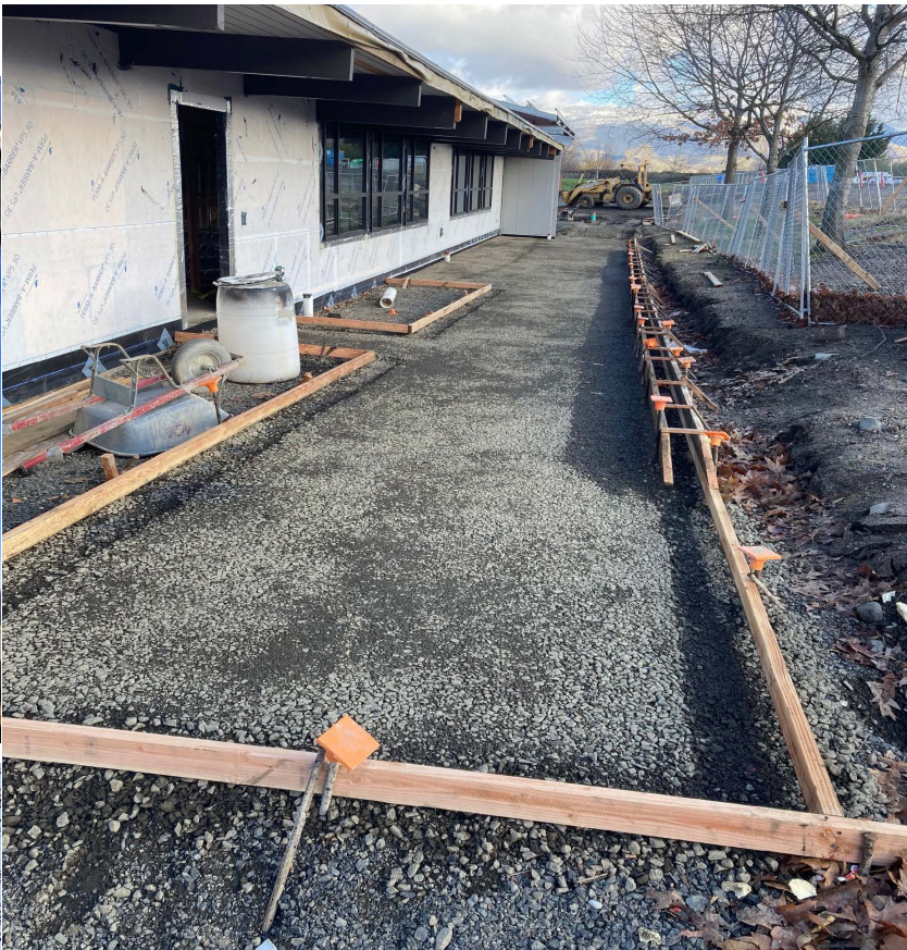
JMOS SIDEWALK FORMED AND READY TO POUR
