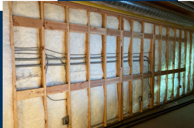
INSULATION IN THE D WING BETWEEN CLASSROOMS
