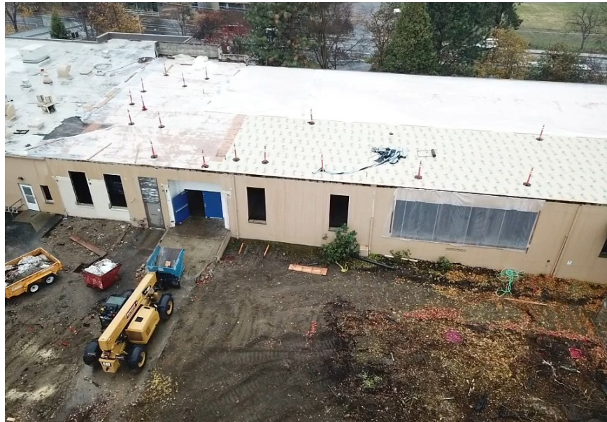
ROOF DEMO AND REPLACEMENT AT RENOVATION
