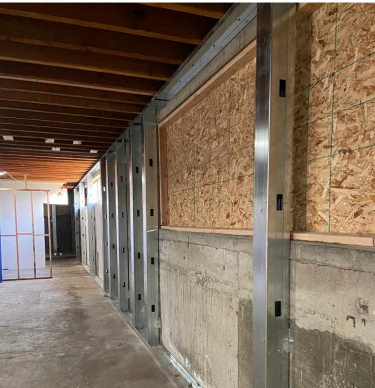
NEW STEEL STUD STRONGBACKS IN BASEMENT
