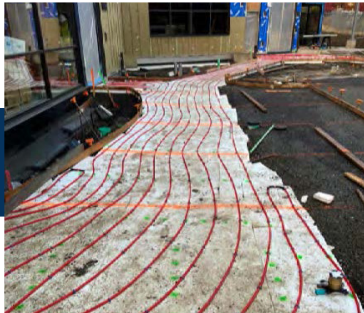
HYDRONIC SNOW MELT LINES THAT WILL BE UNDER
