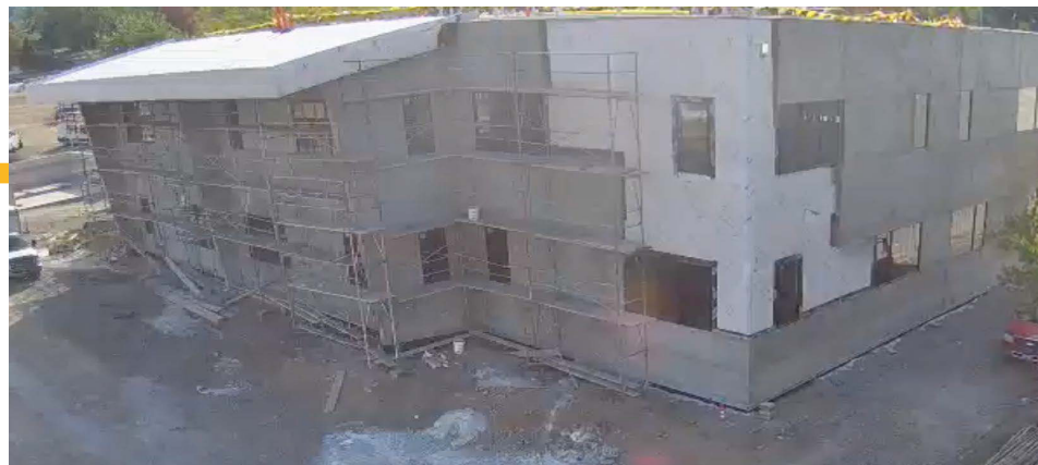
6TH GRADE BUILDING PROGRESS. STUCCO HAS BEGUN.
