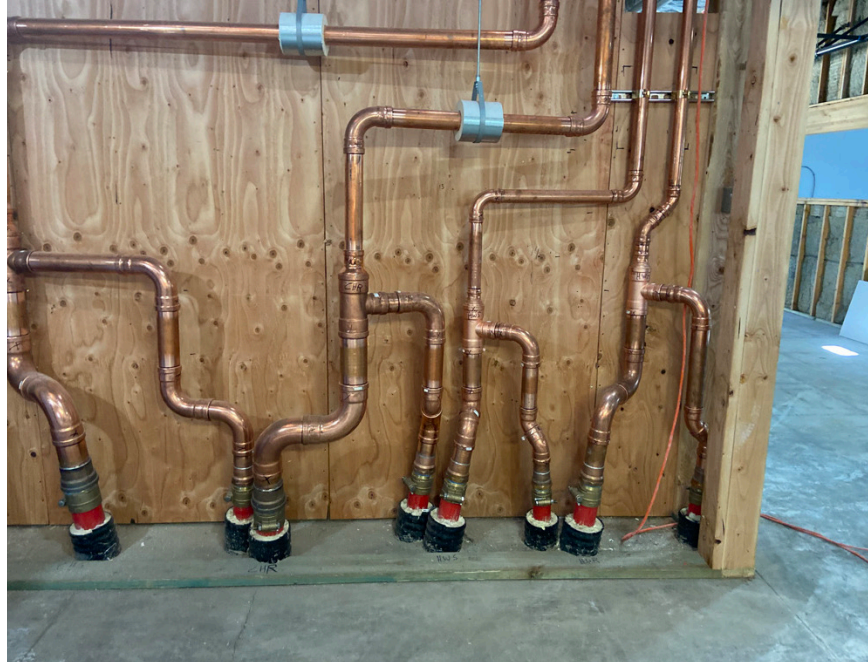
NEW HYDRONIC LINES AT THE NEW BUILDING
