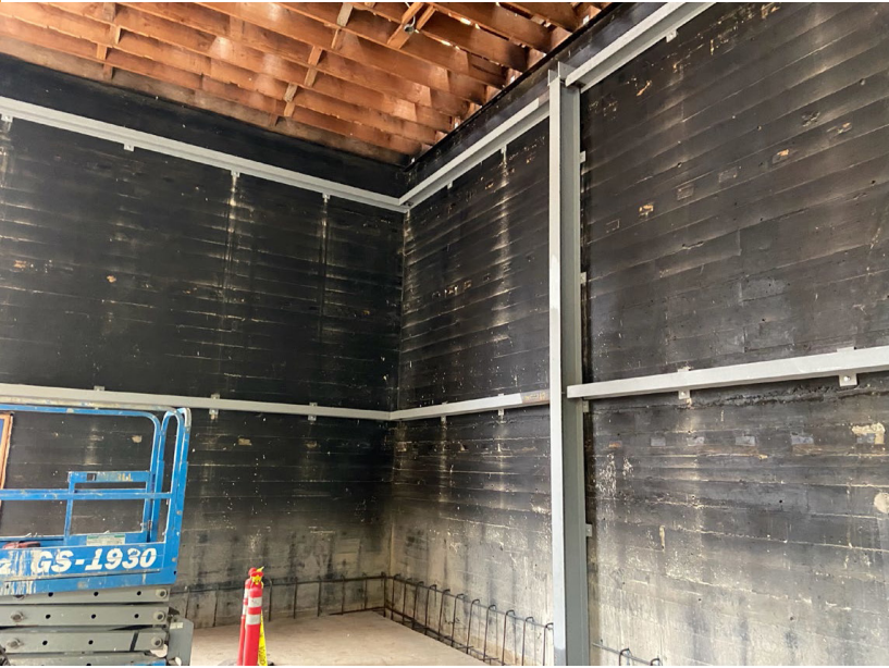
NEW STEEL STRONGBACKS IN CAFETERIA
