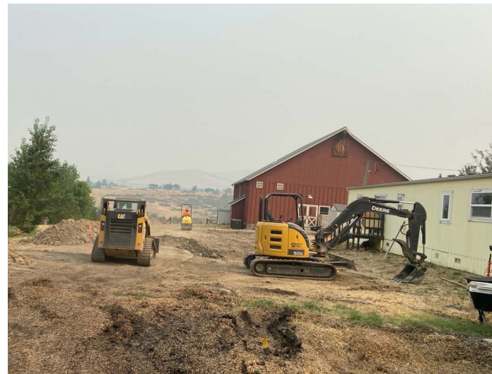
PREPPING THE PAD AND TRENCHING UTILITIES FOR THE NEW MODULAR
