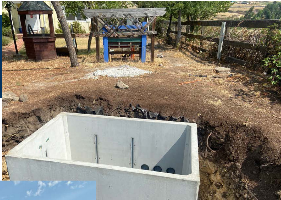
NEW ELECTRICAL SERVICE VAULT
