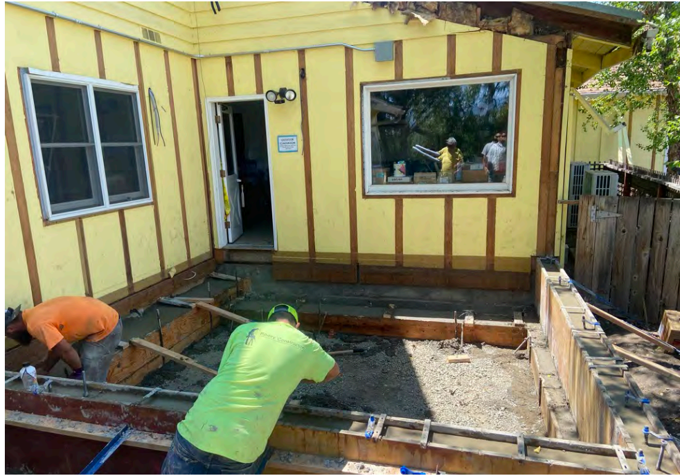
FINISHING NEW STEM WALL FOR HEALTH ROOM
