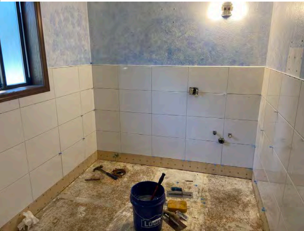
NEW TILE BEING INSTALLED IN BATHROOM
