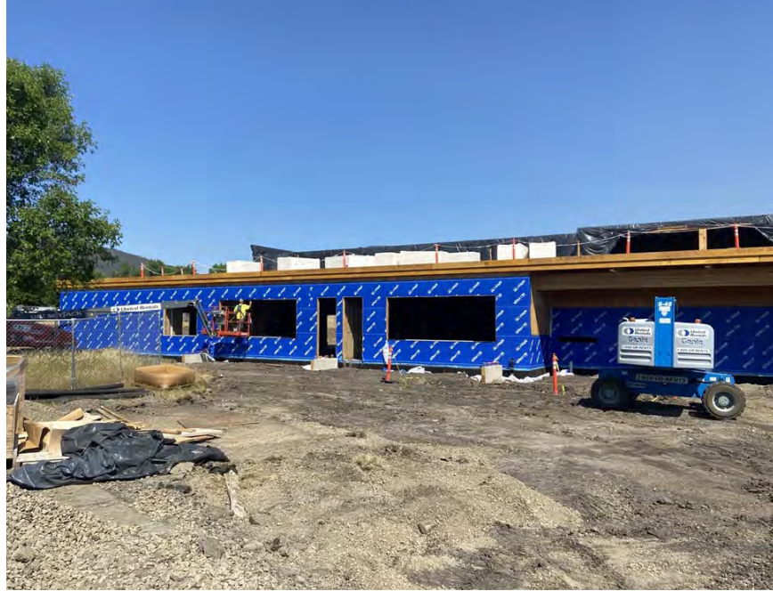
INSTALLATION OF EXTERIOR WRB
