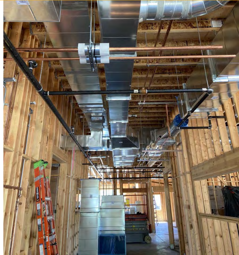
Mechanical ducting for the new HVAC at Helman.
