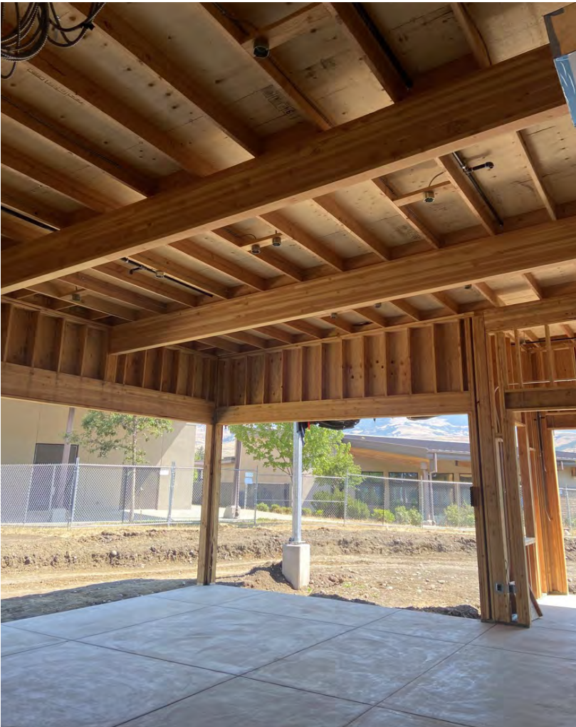
EXPOSED GLULAM BEAMS IN ACTIVITY SPACE
