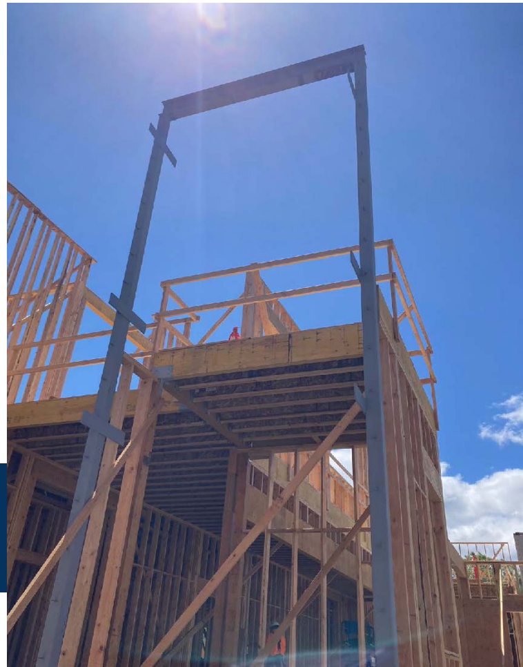
ELEVATOR STEEL SUPPORT AT THE 6TH GRADE BUILDING
