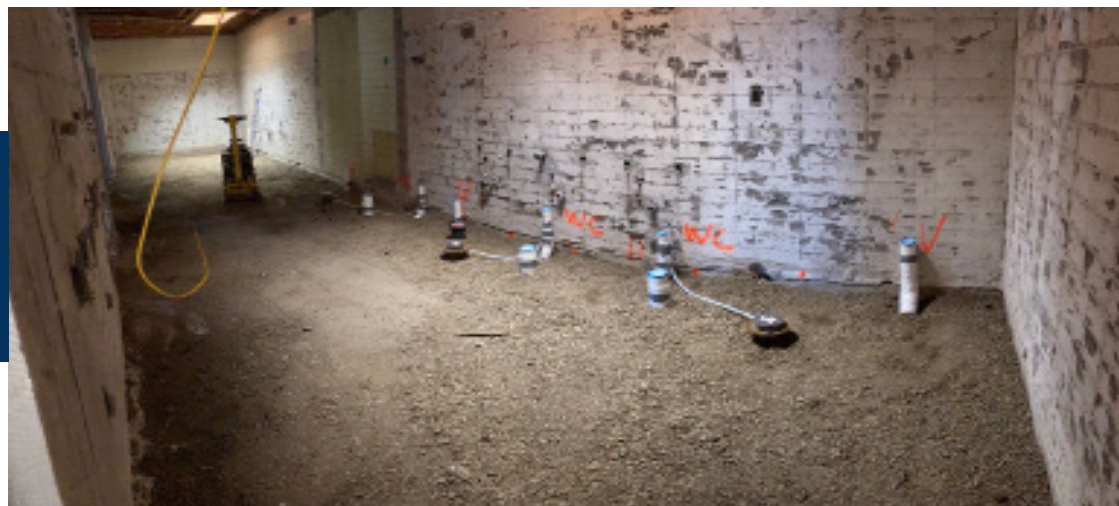
JMOS NEW RESTROOM PLUMBING INSTALLED, BACKFILLED AND READY FOR SLAB ON GRADE
