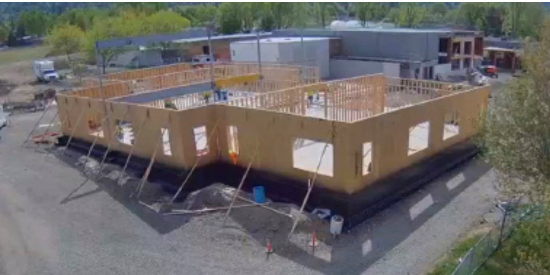
THE NEW 6TH GRADE BUILDING SLAB WITH EXTERIOR WALLS BEING BUILT.
