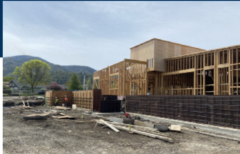
EAST SIDE EXTERIOR WALL FRAMING AND SITE RETAINING WALL
