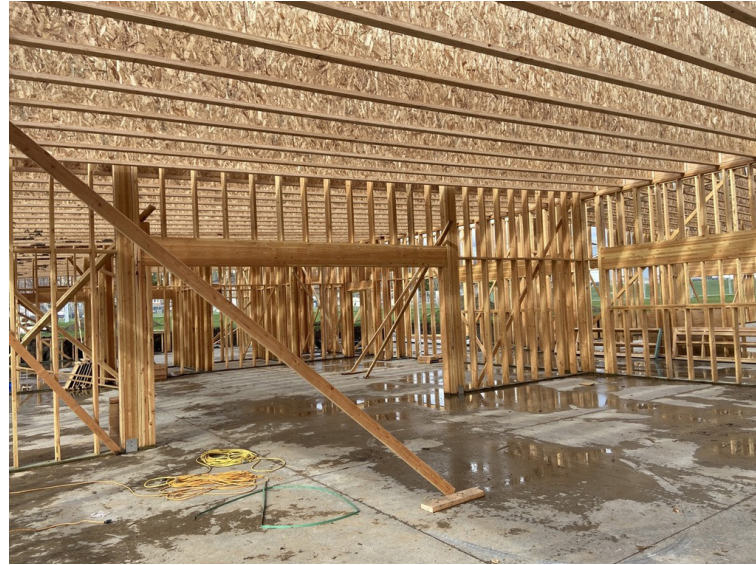
WALLS AND ROOF JOISTS ARE FRAMED
