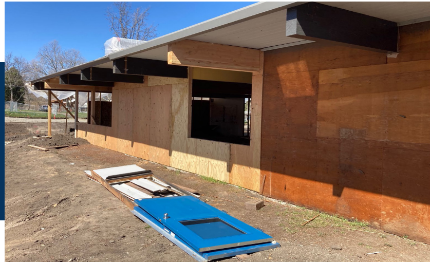
EXTRIOR SUB-SIDING INSTALLATION OUTSIDE ROOMS C126 AND C127
