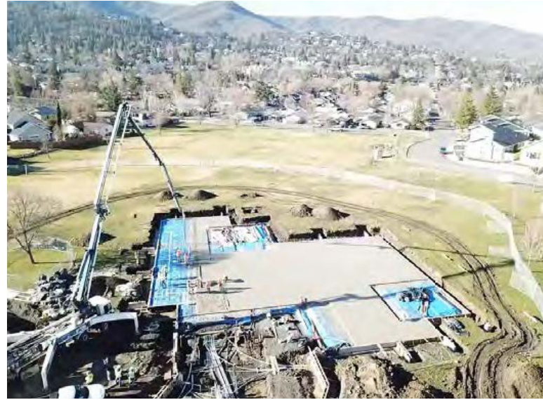
POURING CONCRETE FOR THE WEST SIDE BUILDING
