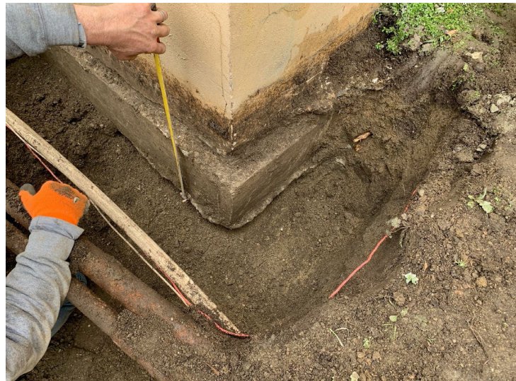
STRUCTURAL INVESTIGATION AT THE EXISTING FOOTING
