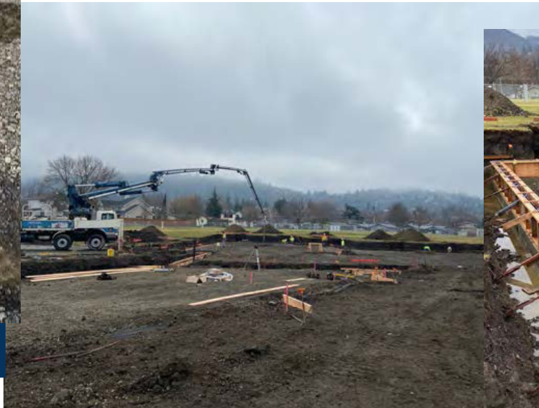
POURING CONCRETE FOR FOOTINGS
