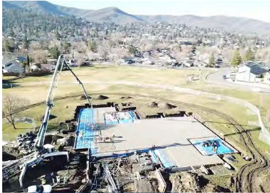
POURING CONCRETE FOR THE WEST SIDE BUILDING PAD
