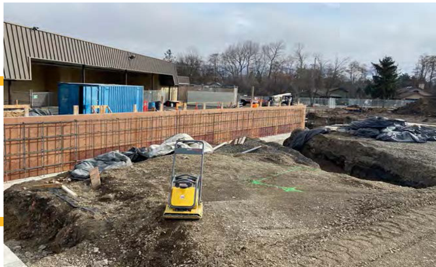
FORMS FOR RETAINING WALL
